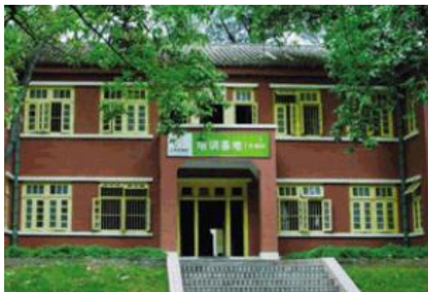
External view of a job training school
